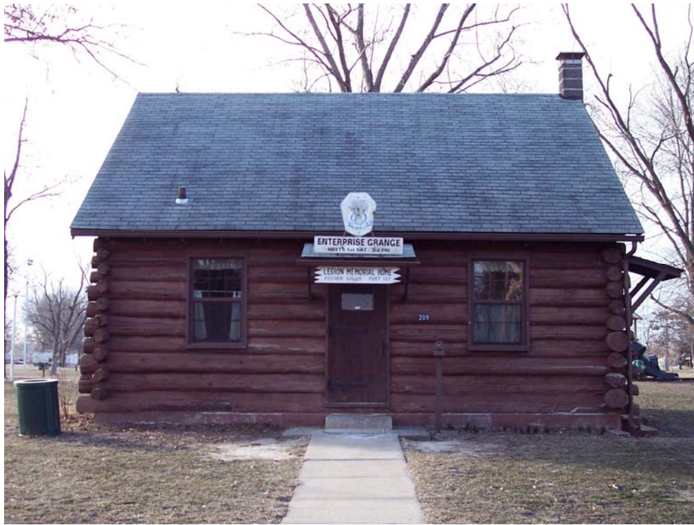
American Legion—Grange Hut top—facing south bottom—facing southwest
