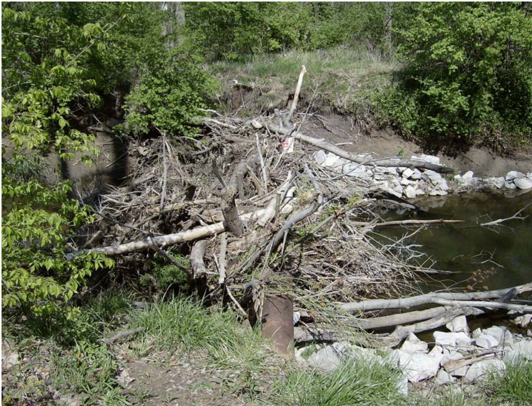
Snag at Braeswood Flyover on Engle Creek – 5/07
