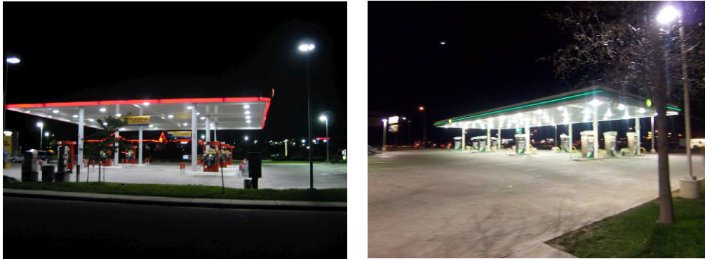
Figure 1 - (Left) Gas station with fully shielded lighting and (right) with ordinary drop lens lighting. The reduced glare and light pollution of fully shielded lighting is required by the Ordinance ( Benya Lighting Design )
