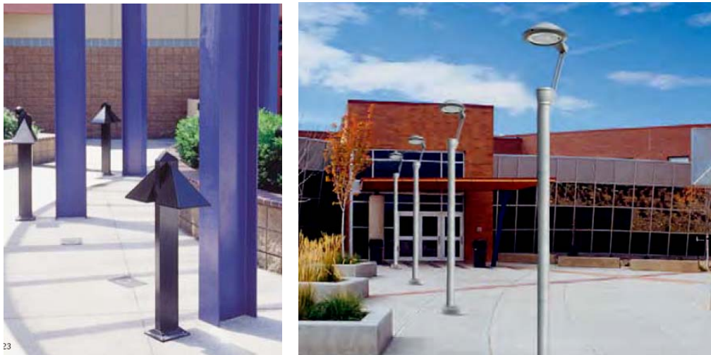
Figure 13- Walkway lighting with ( left ) bollards and ( right ) short pole lights (AAL)
