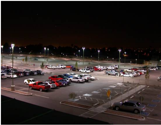
Figure 3 - Every Other Row Option Parking Lot with Fully Shielded Luminaires ( Monrad Engineering, Inc. )
