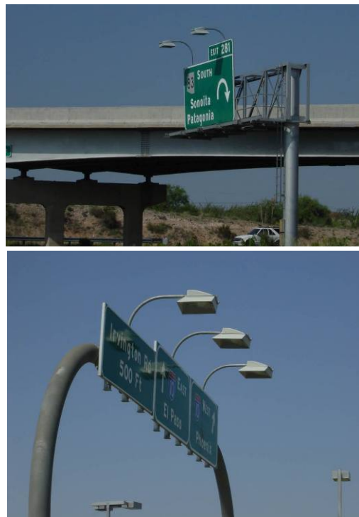
Figure 7 - Top Mounted, fully shielded sign luminaires. Note shielding in the direction of the viewer is critical as well as shielding for potential spill light over the top of the sign ( Monrad Engineering Inc. )
