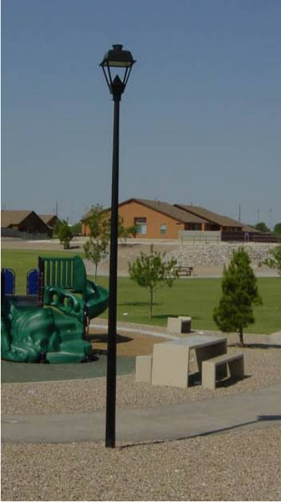
Figure 4 - Fully shielded high performance decorative lighting. Top , flat lens wall lanterns (Lumec); Bottom , post luminaire (GE)
