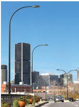
Note that street light design using "full cut off" luminaires is required by the Ordinance. For maximum energy efficiency and minimum maintenance, high pressure sodium lighting is generally preferred. Pole height is not restricted, but as a general rule street lights should be between 20 and 35 feet above grade. Poles are generally mounted 5-6 mounting heights apart along the roadway.
