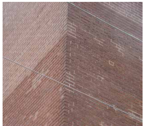
Right: The brick walls at 220 E. State Street are in need of tuck-pointing.
