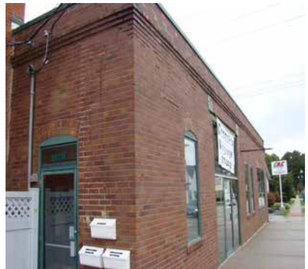
Right: The brick wall at 102 W. State Street is in need of tuck-pointing.
