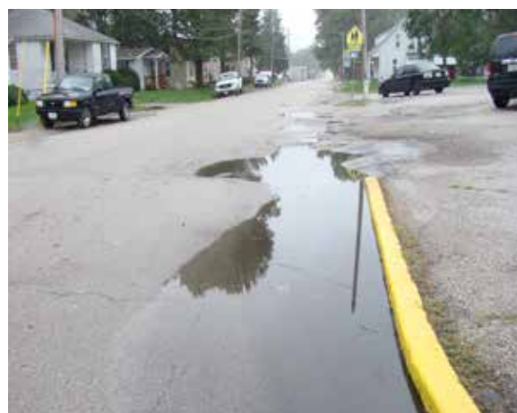
Left: The intersection of W. Fifth Street and Lincoln Avenue has deteriorated pavement and standing water due to inadequate storm drainage.
