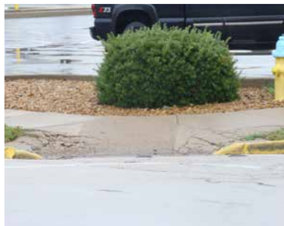
Right: A deteriorated handicap ramp located at the intersection of Lincoln and Third.
