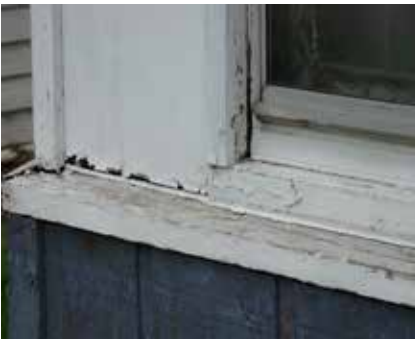
Below: The wood siding and window frame at 112 N. Lincoln Avenue are deteriorated.
