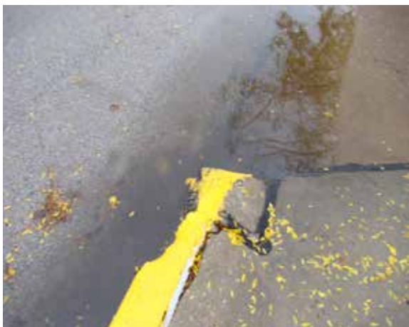
Left: Deteriorated curbing along Lincoln Avenue. Note: standing water due to inadequate storm drainage.
