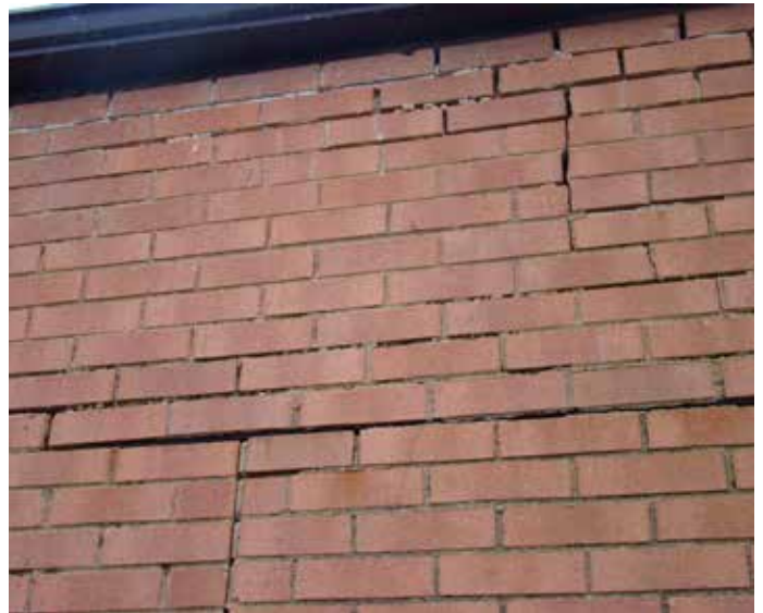
Above: The rear of the eastern building located at Southview Plaza is in need of tuck-pointing.
