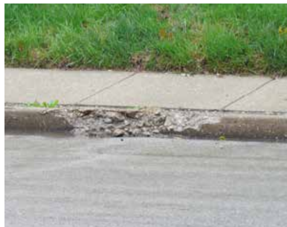
Right: Deteriorated curbing along S. Lincoln Avenue.
