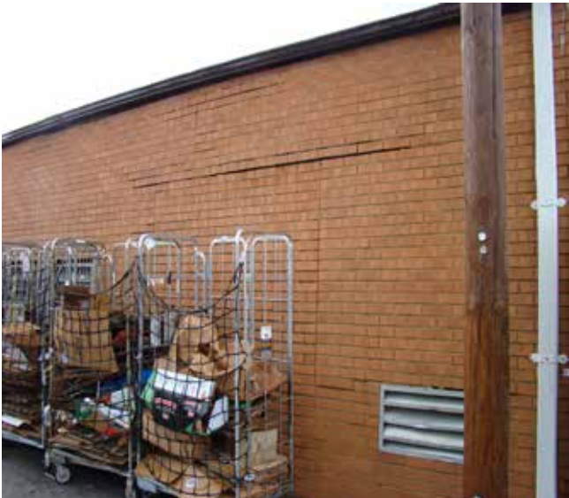
Above: The rear of the eastern building located at Southview Plaza is in need of tuck-pointing.
