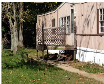
Above: A rotted wood porch on the front of one of the mobile homes at Rock Springs Estates.
