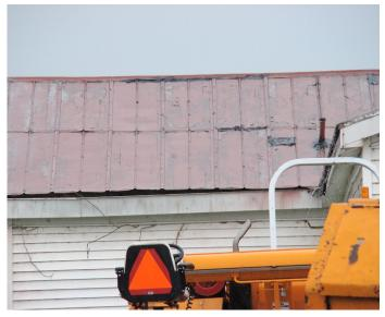
Above: The corrugated metal roof at 201 Scott-Troy Road is deteriorated.
