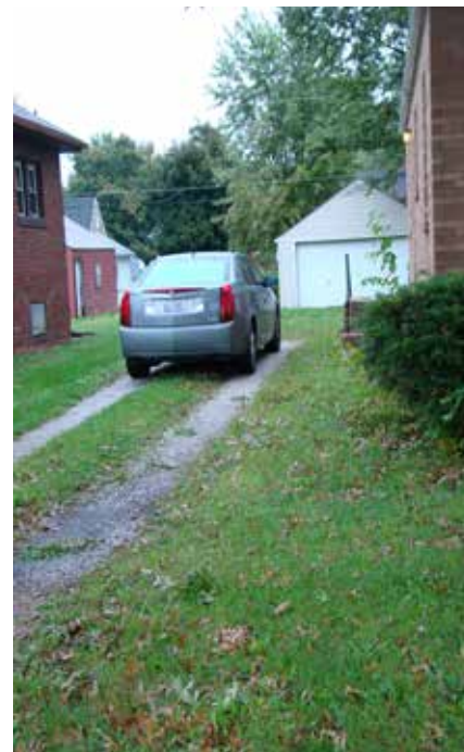
Below: A deteriorated gravel driveway located at 708 S. Lincoln
