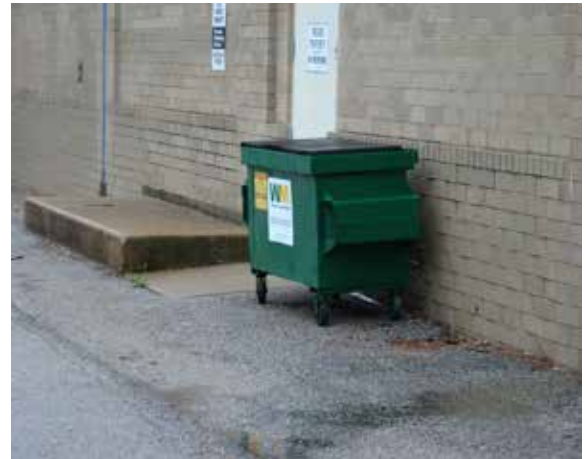
Right: An un-screened dumpster behind 502 S. Lincoln Avenue.
