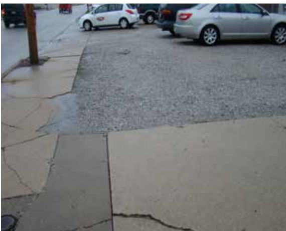
Left: The entire lot for 510 S. Lincoln is covered in parking lot. Note: drivers must back out onto S. Lincoln Avenue.
