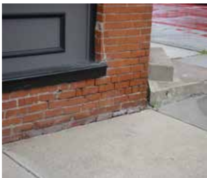
Above: Sections of 104 S. Cherry are in need of tuck-pointing and are deteriorated.
