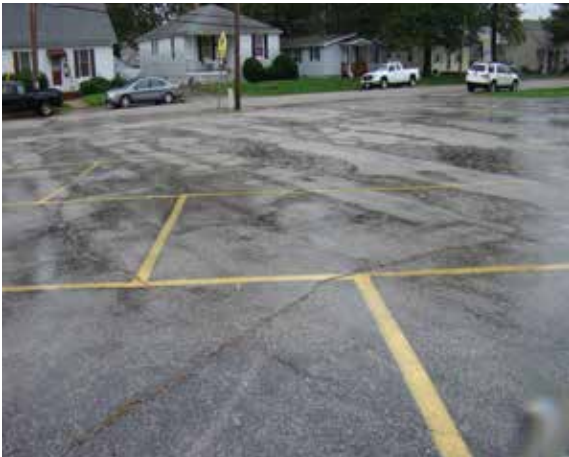
Left: The entire lot for 403 S. Lincoln has been paved.
