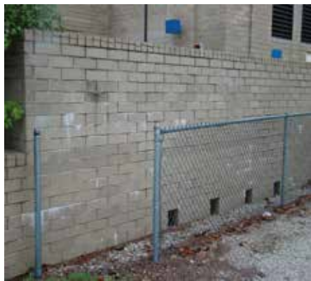
Above: the brick wall located at 502 S. Lincoln Avenue is in need of tuck-pointing.
