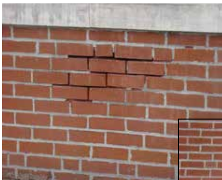
Above & Right: Sections of 111 W. Second are in need of tuck-pointing.
