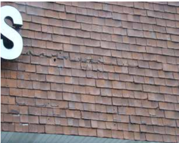
Left & Right: Deteriorated shingles on a building at Southview Plaza.
