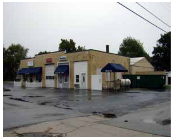
Right: The entire lot for 102 S. Vine has been paved.
