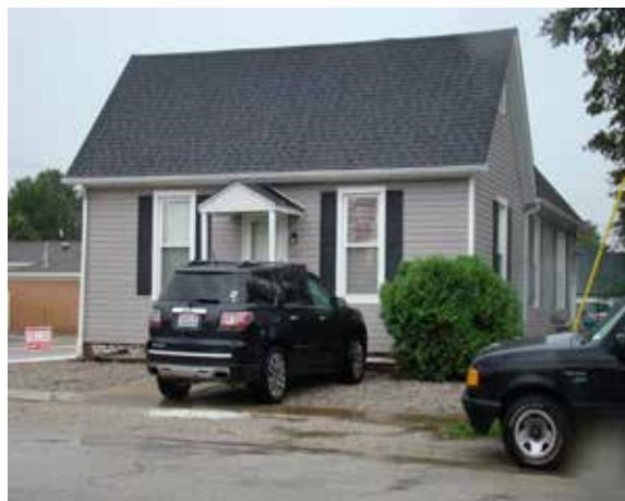
Right: 101 W. Fifth Street has a parking lot that requires drivers to back out onto the street.
