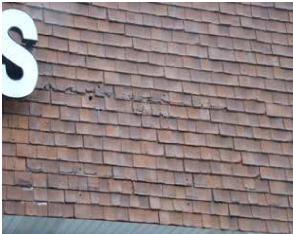
Left & Right: Deteriorated shingles on a building at Southview Plaza.
