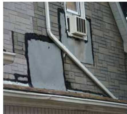
Below: Deteriorated asphalt siding on 304 S. Lincoln Avenue.
