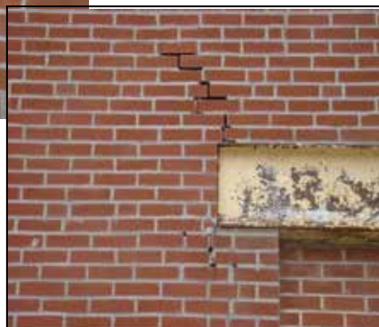
Above & Right: Sections of 111 W. Second are in need of tuck-pointing.
