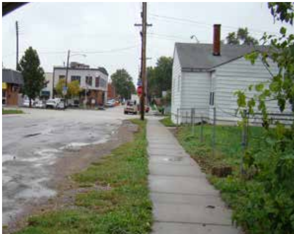
Left: The pavement along N. Cherry Street is deteriorated.
