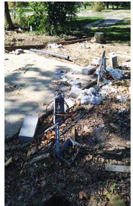
Above: Wiring and building debris at a vacant mobile home pad.
