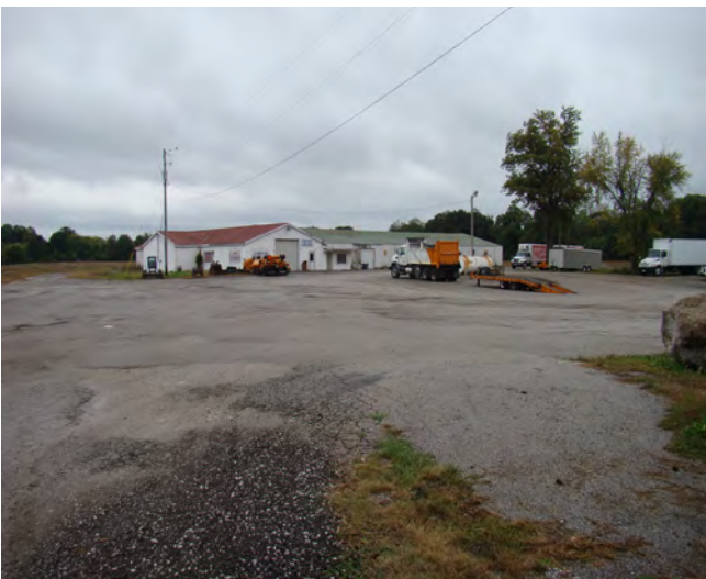
Above: The parking lot at 201 Scott-Troy Road is deteriorated. Left: Tractor-trailers and other heavy equipment stored at 201 Scott-Troy Road. This property is directly adjacent to a residential subdivision located across the street to the east.
