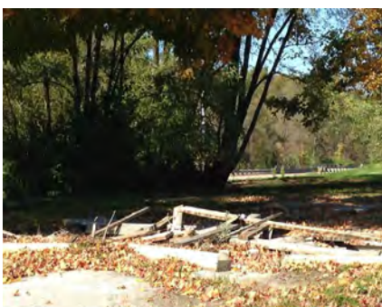
Below: Building debris on a vacant lot at Rock Springs Estates.
