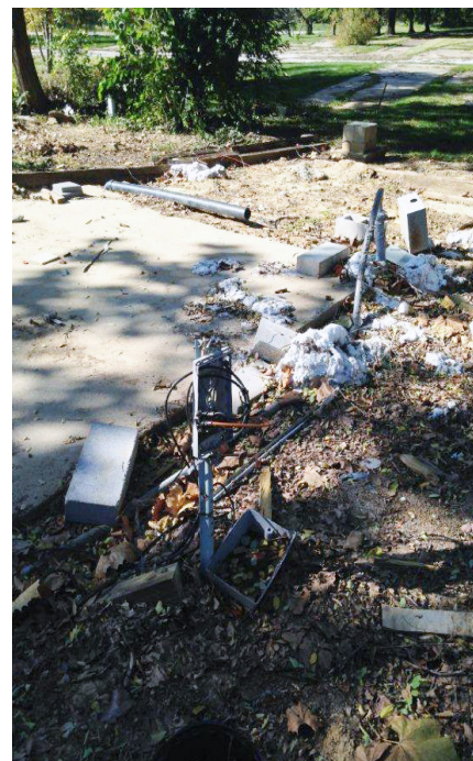
Above: Wiring and building debris at a vacant mobile home pad.
