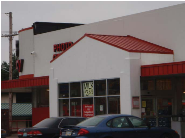
Roof design contains no eaves on projection
