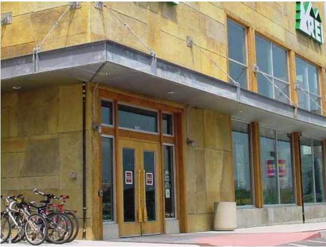
Metal awning provides shade and durability
