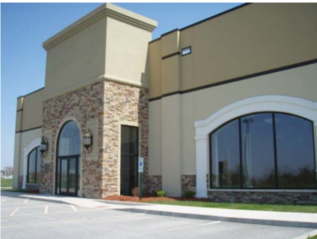
Entry is defined with change in material and projection
