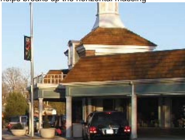
Arcade for pedestrians is formed from roof eaves
