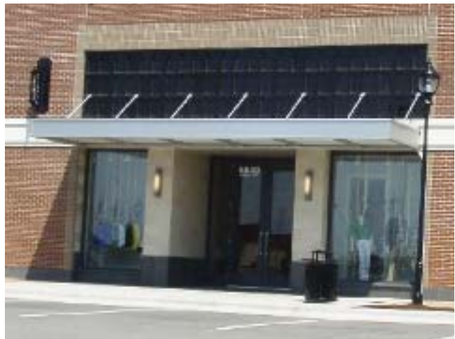
Metal awnings help define the entryway and provide protection from the elements
