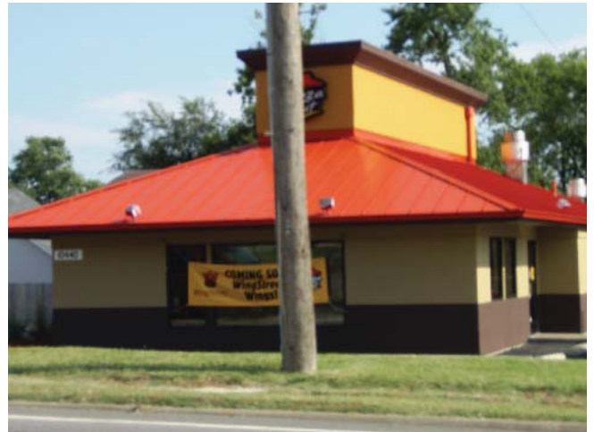
Roof design combines roof types unnecessarily
