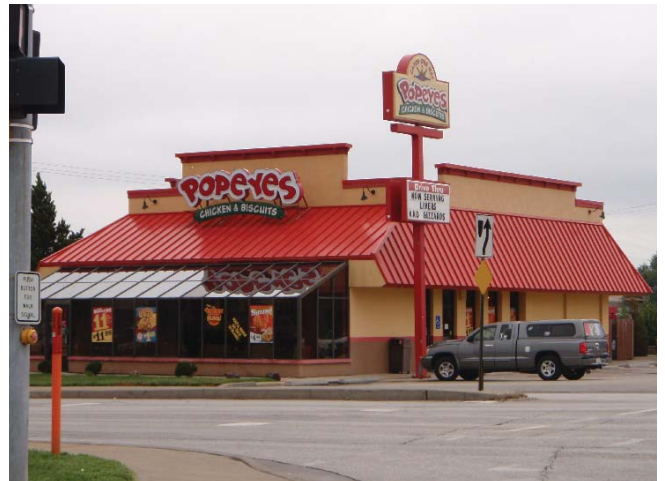
Roof design includes too many roof forms and slopes
