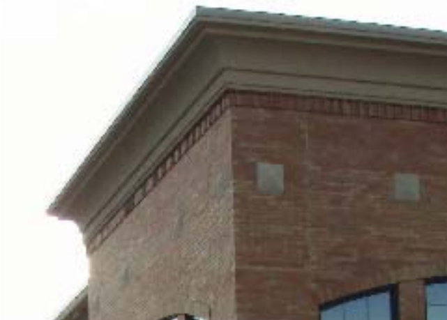
Cornice wraps the corner on street facing façades
