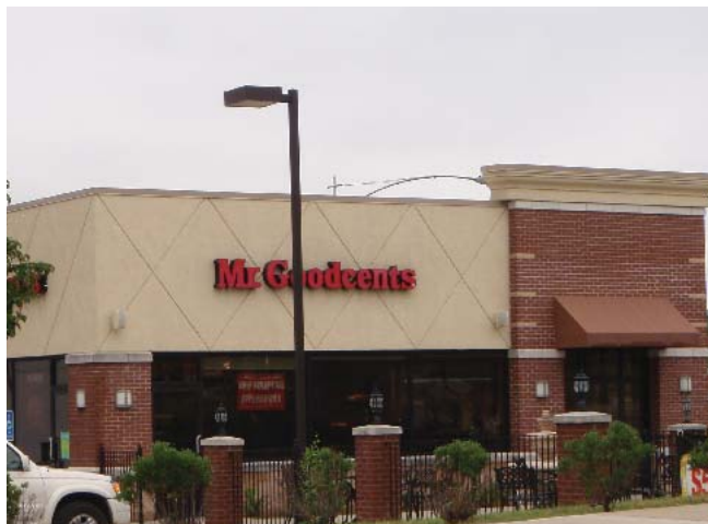
Parapet does not extend across all street facing façades
