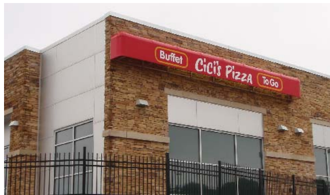
Awning is too high and small to provide cover for pedestrians
