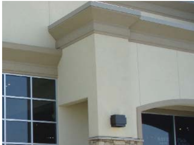
Cornice wraps all the way around projections
